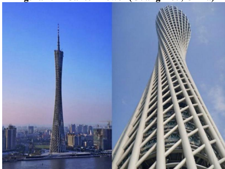
Figura 2.2 - Canton Tower (Guangzhou, China)
