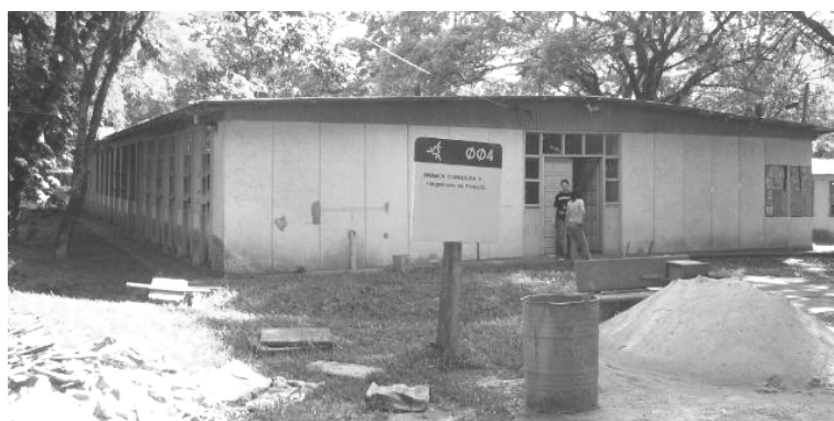
Foto 6.1.12 – Bloco 004 (Administrativo DHI-NIE-DCS-Propae/Pread/PPE) [2005].
