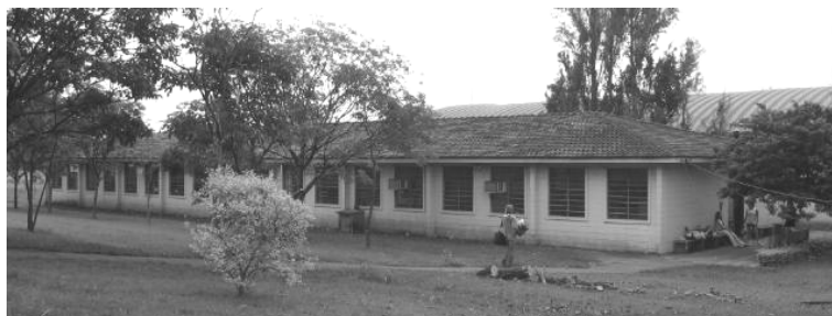
Foto 6.2.23 – Bloco M06 (Administrativo DEF) [2005].
